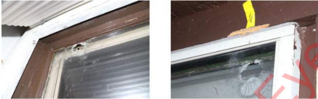
Figure 33 (WSCL R22-3576-1_LMN_IMG_0765.JPG and WSCL R22-3576-1_LMN_IMG_0958.JPG) Penetration in Upper East Corner of Upper Half of Southeast Window in Southwest Bedroom (Left: View from the Interior | Right: View from the Exterior)
